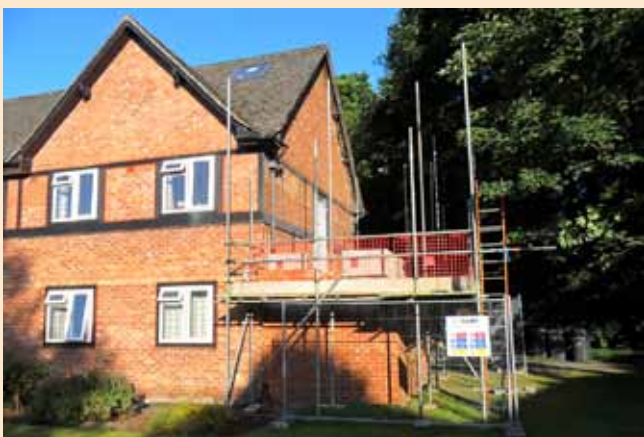
The "Tower" under construction
